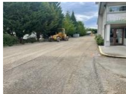
Parking lot regrading in progress
